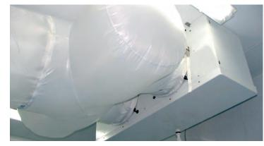
VGT option used to fasten the textile duct (not supplied).
