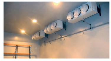
VPM option - Shell / air stream deflector (streamer) + flexible defrost sleeve Avoid circulation of hot air during defrost cycles. Reduction of defrost cycle time for energy saving.
