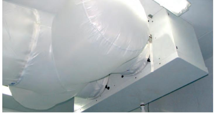
VGT option used to fasten the textile duct (not supplied).
